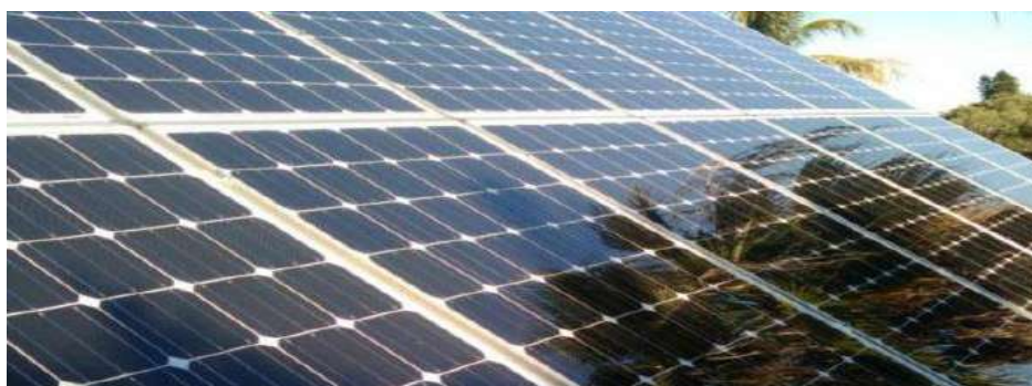
Figure: Tree shadow over modules
