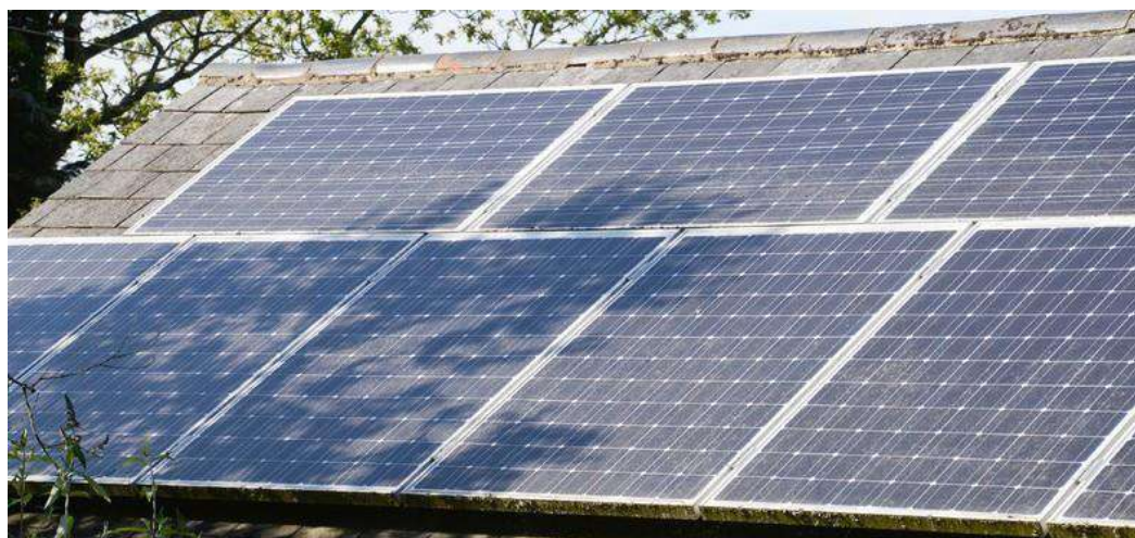
Figure: Shading on PV Modules
